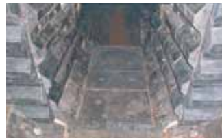
Inlet Chutes, with water added and carefully lined with rubber.
