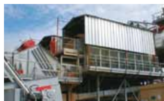
Complete Installations Pre-separation, De-mudding, After Washing and Dewatering.
