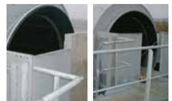
Service Access Bridge for internal maintenance of e.g. lining.
